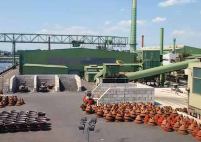
View of the new North Plant warehouse
