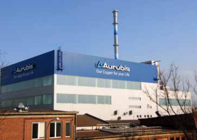
The new anode slime processing building
